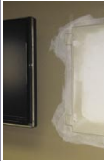
STEP 3: APPLY JOINT COMPOUND AND SAND UNTIL SMOOTH
