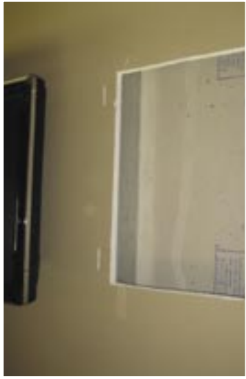
STEP 1: RUN THE WIRE AND CUT THE HOLE INTO THE WALL
